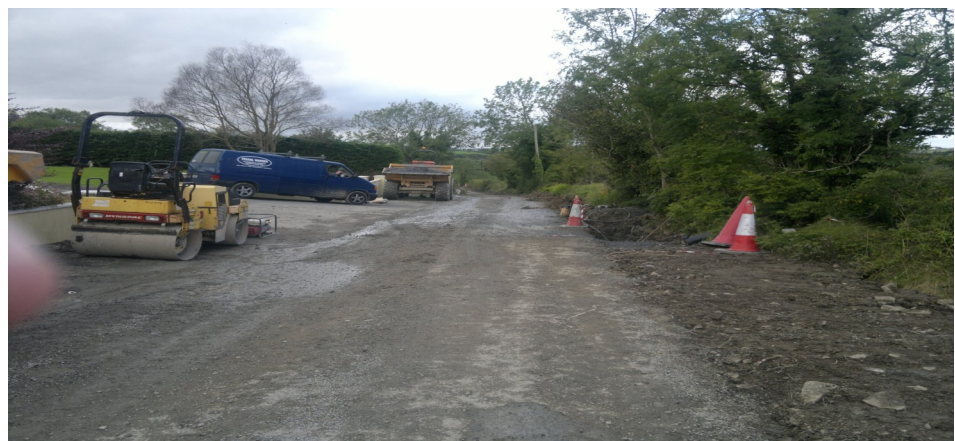
Upgrade work being carried out in Dromadrehid by Mainland Construction.
